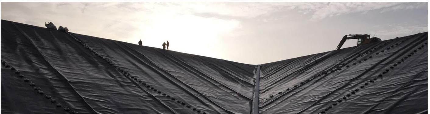
PTES heat storage basin or pit is lined with the Solmax high-temperature geomembrane.
